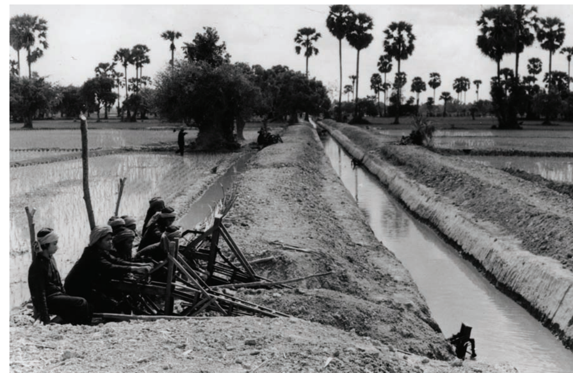
Khmer Rouge Female Mobile Unit pedaling to transport water for irrigation. (Documentation Center of Cambodia Archives)
