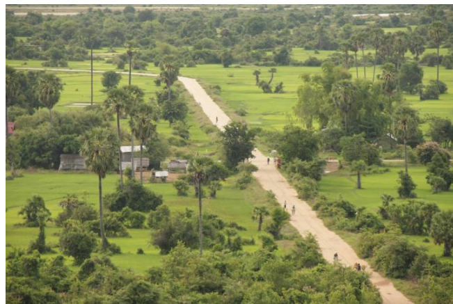
Road to Kampong Chhnang Airport
