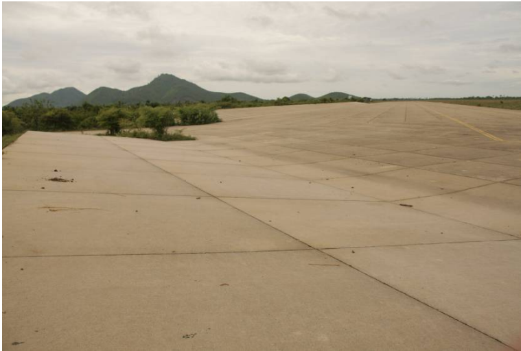
The running road of Kampong Chhnang airport
