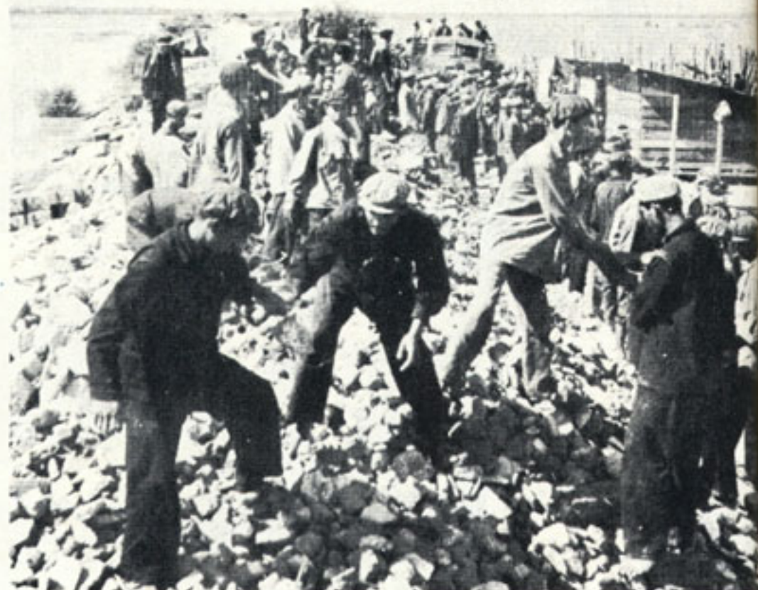
Reinforcement work on the Prek Phneou dyke north of Phnom Penh.
