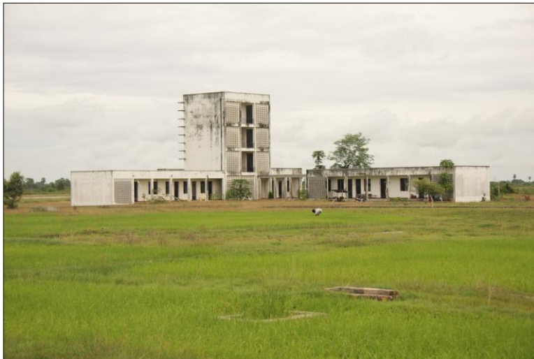
Control tower at incomplete Kampong Chhnang airport
