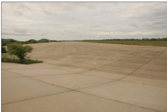
Runway at Kampong Chhnang airport
