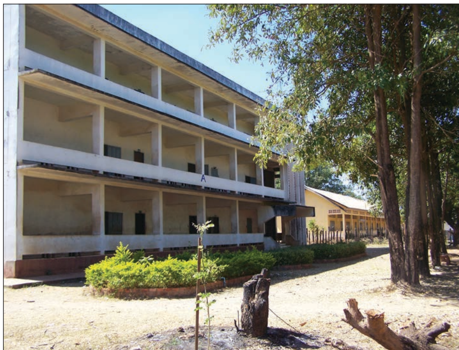
Anlong Veng High School: One of the main buildings was built by Ta Mok, 2012. Photo by Christopher Dearing.
