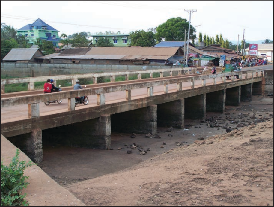
Ta Mok Bridge, 2012, Photo by Christopher Dearing.
