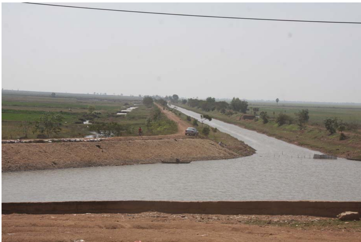
Irrigation System at Trapeang Thma Dam
