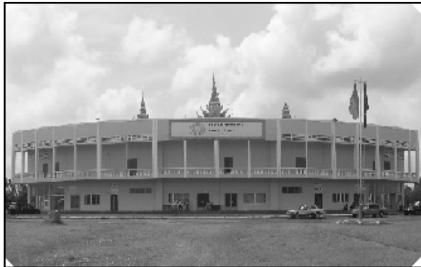
The ECCC courtroom is located on Route 4, just behind the National Army Headquarters, Phnom Penh.
