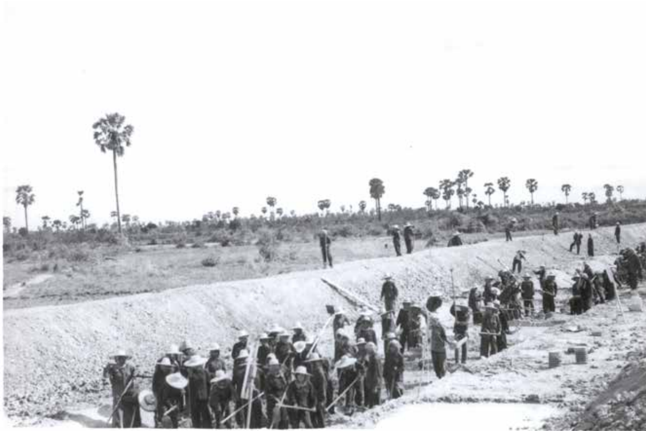
Cambodian people digging the dam in the suburb of Phnom Penh during the Khmer Rouge regime. All people were obliged to work during the regime. The Khmer Rouge regime compelled large portions of the population to conduct manual labor on a daily basis in order to increase the country's production of rice.
